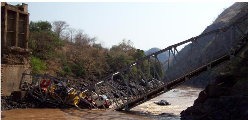
crashed into the girder upper bracing causing the whole structure to collapse. The traffic had to be diverted back onto the concrete girder with the same load restriction and a reduced carriageway width. The heavier freight had to be rerouted through Nekempt increasing the trip by 150 km along smaller and un-paved roads with severe damage to the country economy.
