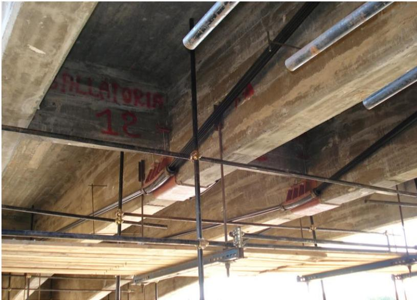
resin and small fasteners to hold them in place before the resin hardened and the prestressing force pushed them against the concrete section. Deviation pipes were installed inside holes previously bored into the diaphragms with man held equipment.
