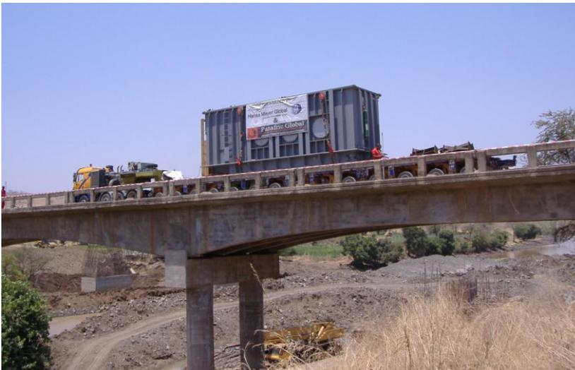
load were conducted so as to simulate the transformer crossing. The bridge was loaded with four 40 tons trucks located so as to maximise shear and hogging moments close to the central piers. The bridge did withstand this test loading although displacements clearly indicated a non linear response due to some sort crack activation or re-activation. Elastic recovery was satisfactory though and therefore crossing of the transformers was given the go ahead.
