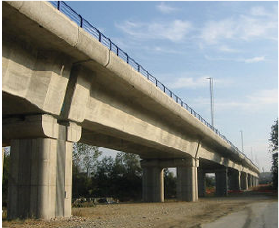
Fig 10 The finished viaduct (Chivasso)
