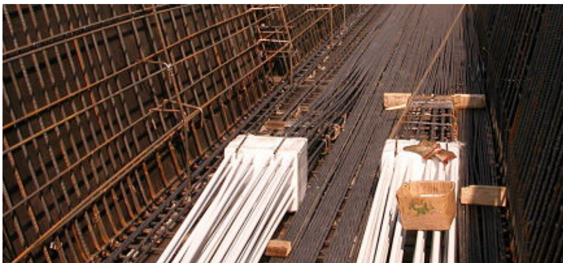
Fig. 4 The sheathed strands and the cutting boxes
