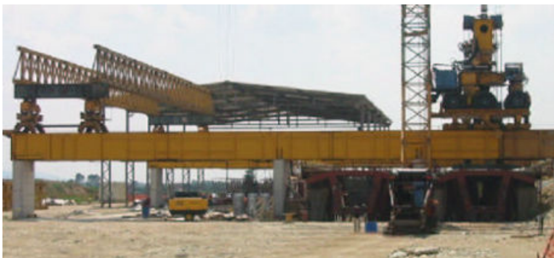
Fig. 7 Prefabrication yard at Chivasso
