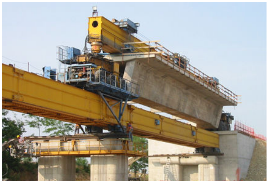
Fig 9 Launching with the under bridge
