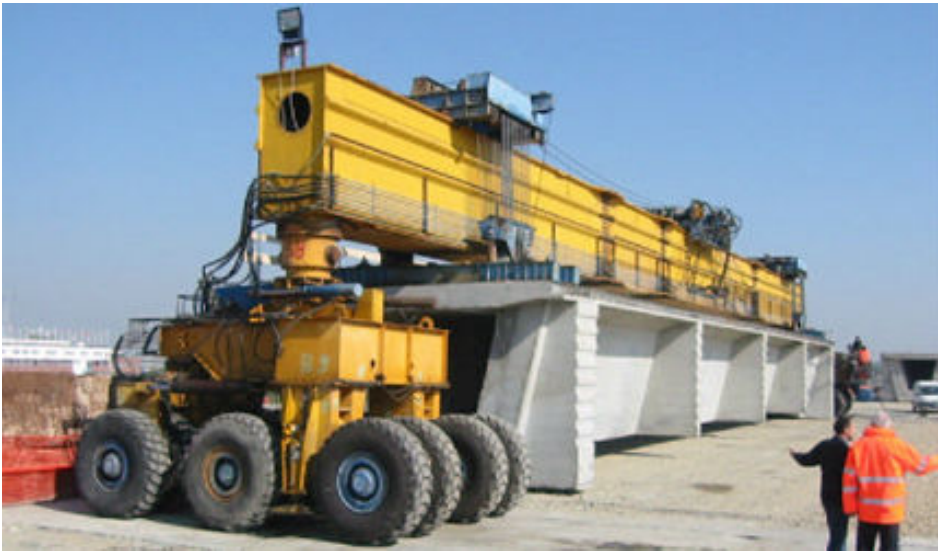
Fig 8 The truck crane
