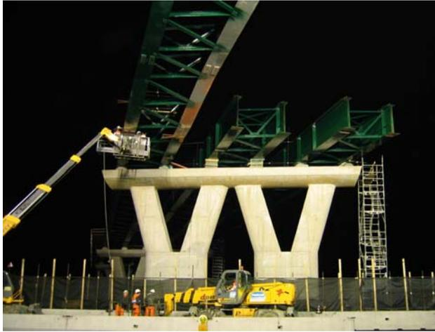
Photo 1 – Lifting the SS11 overpass into place
