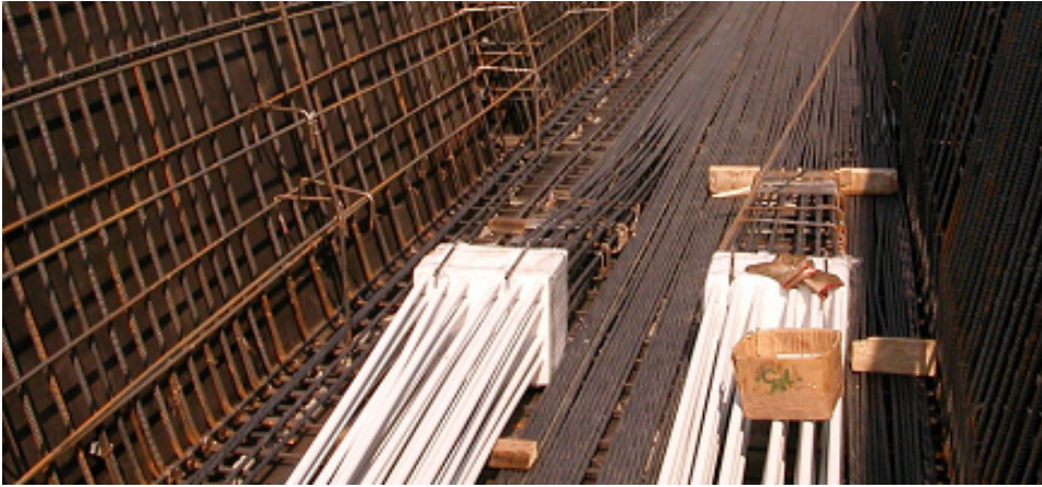
Photo 2: The sheathed strands and the cutting boxes
