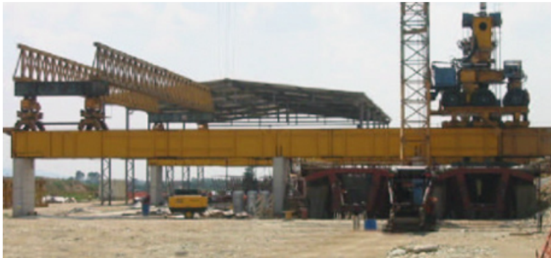
Photo 3: Prefabrication yard at Chivasso
