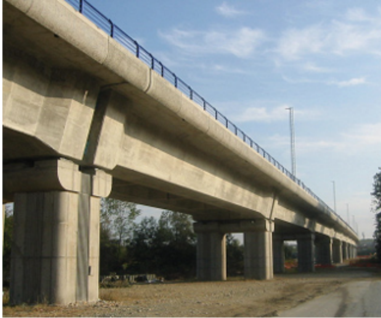
Photo 6: The finished viaduct at Chivasso
