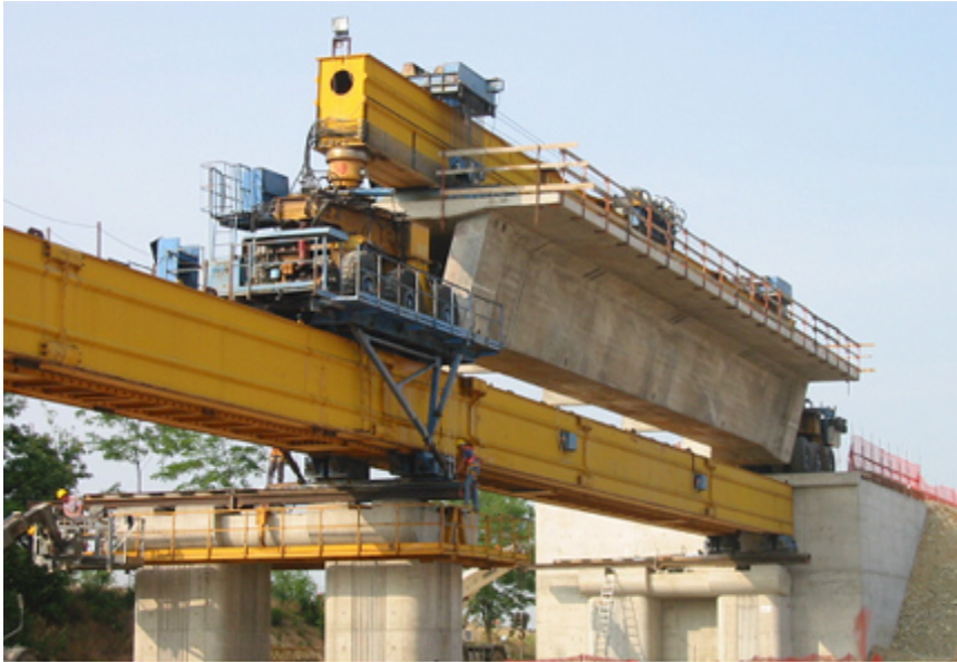
Photo 5: Launching with the under bridge
