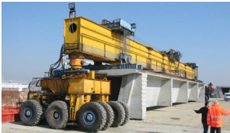
Photo 4: The truck crane
